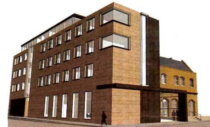
A wall of brass greets visitors at the new entrance to Britton Street. The Albion Place elevation is clad in mainly York stone.
