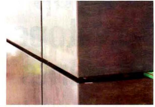
The brass panels' patination is never identical but together they create a uniform impression.
